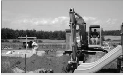
Daryl and Marcia Worcester and the Big Excavator!
